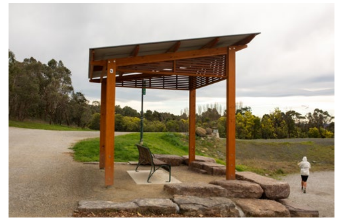
figure 9 Existing shelter and seating
