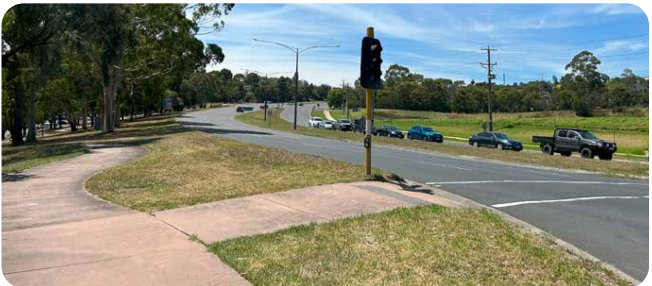
Maroondah Highway is a significant road corridor.
