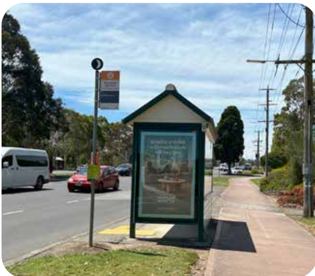
Bus stop located along Maroondah Highway
